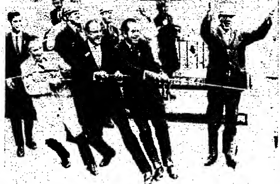
PRESIDENTIAL PULL—Saturday, President Nixon visited the construction site for the multi-million-dollar Libby dam...
